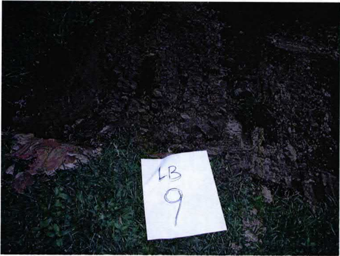
Laurel Bay # 9/ During excavation
