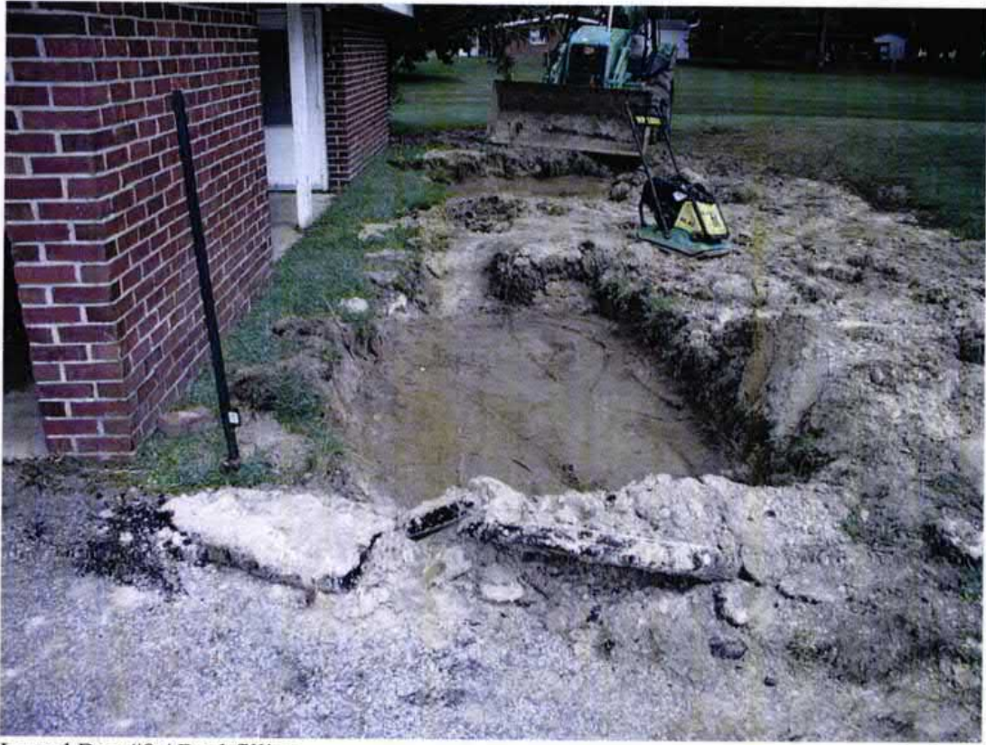
Laurel Bay #9 / Backfilling
